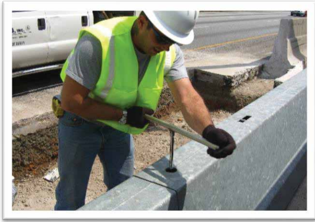
Security Nut Installation
